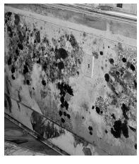
ing and, if possible, use speed drying equipment and moisture meters. Regrowth may signal that the material was not dry enough or should be removed.
