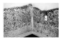
A flood-damaged home needs special care to remove mold safely and effectively. Mold begins to grow on materials that stay wet longer than two or three days. The longer mold grows, the greater the health hazard and the harder it
