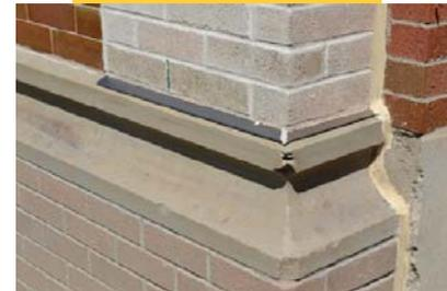
4. All through wall flashing shall be 16 oz. minimum copper or equivalent fabric coated copper. Other metals, vinyls and plastics shall not be used.
