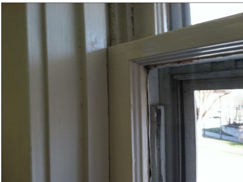
Interior and exterior window frame, trim, sill and header all painted with lead based paint.
