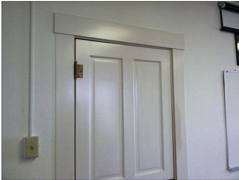
White door trim and door with lead based paint.
