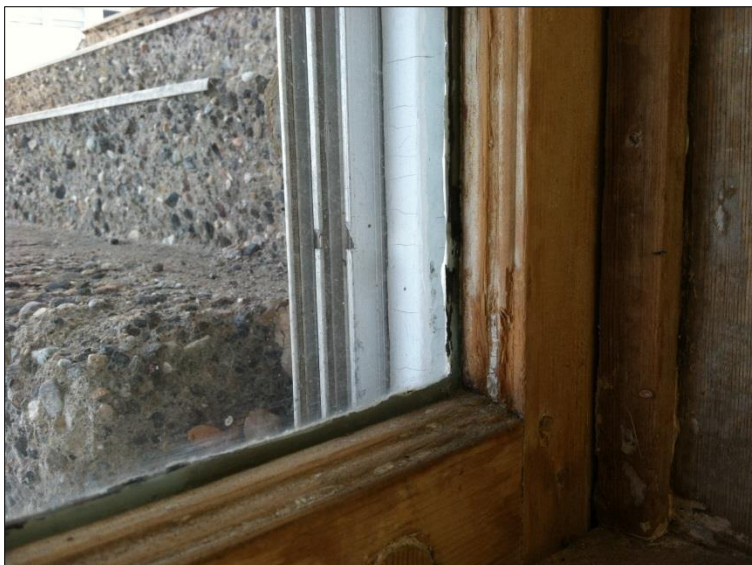
Basement Interior Windows-stripped of lead paint. Exterior window frame remains with lead based paint (white).
