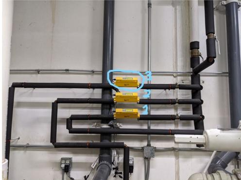
Figure 10: Flowmeters used to measure inlet flow
